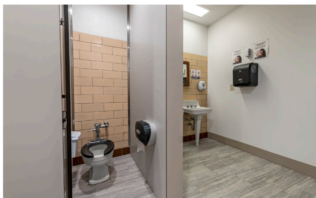
All-gender restrooms designed for the School District of Clayton. The district installed these new restrooms to protect student safety by reducing bullying. Photographs courtesy MR & Associates, Inc.
